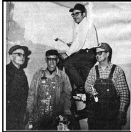
After the fire repairs.
