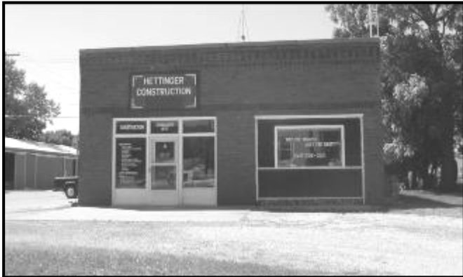
HETTINGER CONSTRUCTION 119 E. Sale St.
