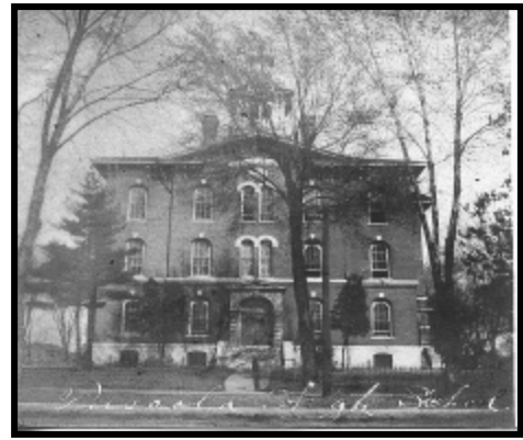
The Union School was completed in 1871 at a cost of $42,000. It was a three-story building of brick with a stone foundation.
