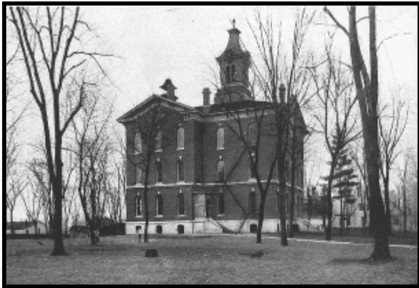
The Union School had 12 rooms above the basement, 10 classrooms, assembly room, superintendent's office and laboratory. The entire third floor was occupied by the high school students.
