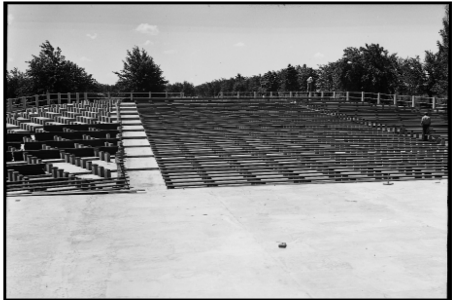
The photo on the right, taken in 1939, is of the amphitheater in the north end of Ervin Park being built by WPA labor. Many good times were had in this arena during the summer months. Picture courtesy of Pettitt Photo Service
