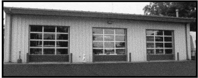
Tuscola Fire Department South Branch Located on the corner of Main and Pinzon Streets.
