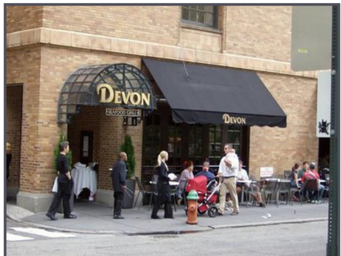
Building Projections - Awnings or canopy structures help define the building entrances and provide visual interest along the street frontage.
