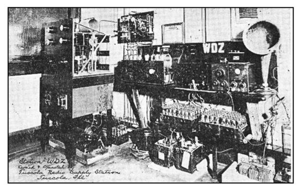
This was the second of four transmitters used by the station. The 50-watt transmitter shown was used from 1923 until 1931. This station used A and B storage batteries. This was before electronics experts had learned how to convert alternating current into direct current.
